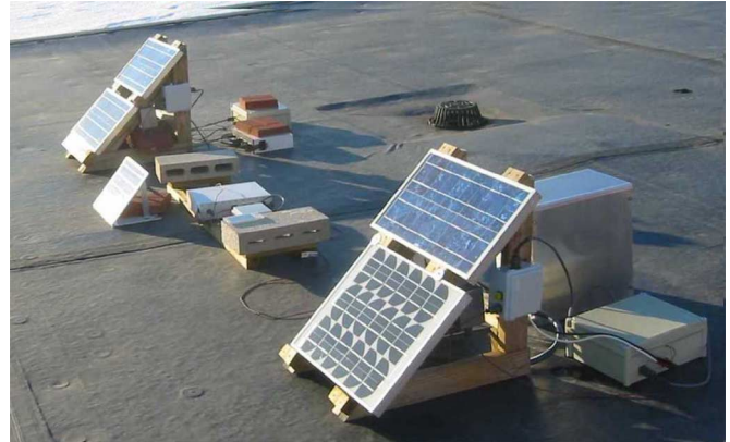
Fig. 10. Demonstration units with a variety of solar panel and energy storage configurations, deployed for testing in Champaign, IL.
